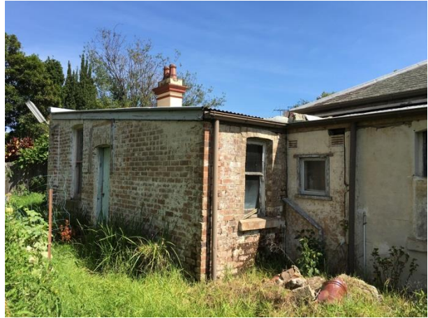
PICTURE 6 – EXTERNAL VIEW OF REAR SOUTHERN FAÇADE.
