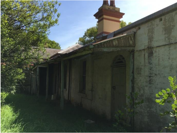
PICTURE 5 – EXTERNAL VIEW OF WESTERN FAÇADE.
