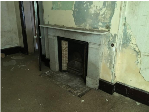
PICTURE 7 – INTERNAL VIEW OF PRINCIPAL ROOM.
