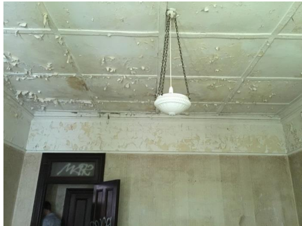
PICTURE 8 – INTERNAL VIEW OF PRINCIPAL ROOM AND TIMBER JOINERY.
