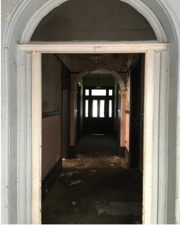
PICTURE 11 – INTERNAL VIEW OF CORRIDOR.
