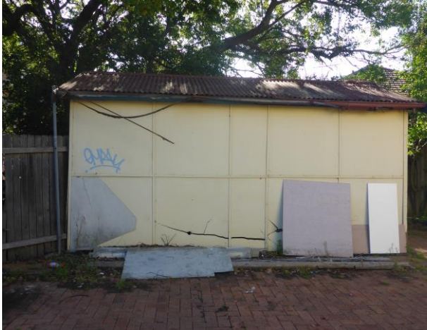
PICTURE 19 – EXTERNAL VIEW
