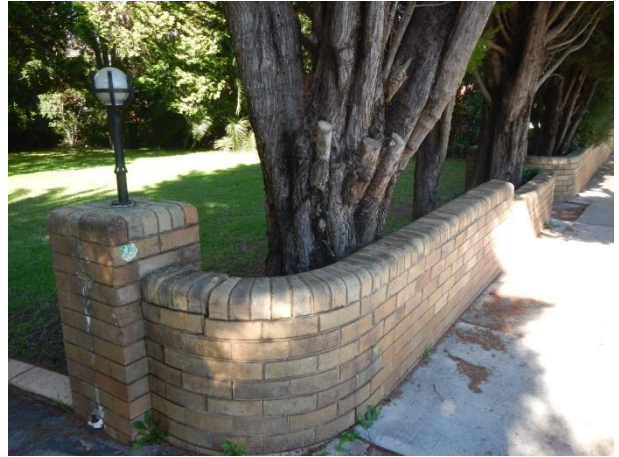
PICTURE 26 – FRONT FENCE
