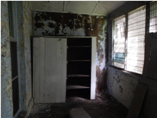
PICTURE 13 – INTERNAL VIEW OF EXISTING INFILLED WESTERN VERANDAH.
