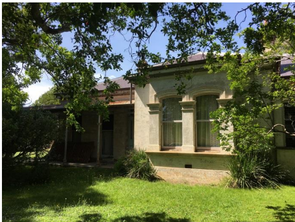
PICTURE 1 – PRINCIPAL NORTHERN FAÇADE.
