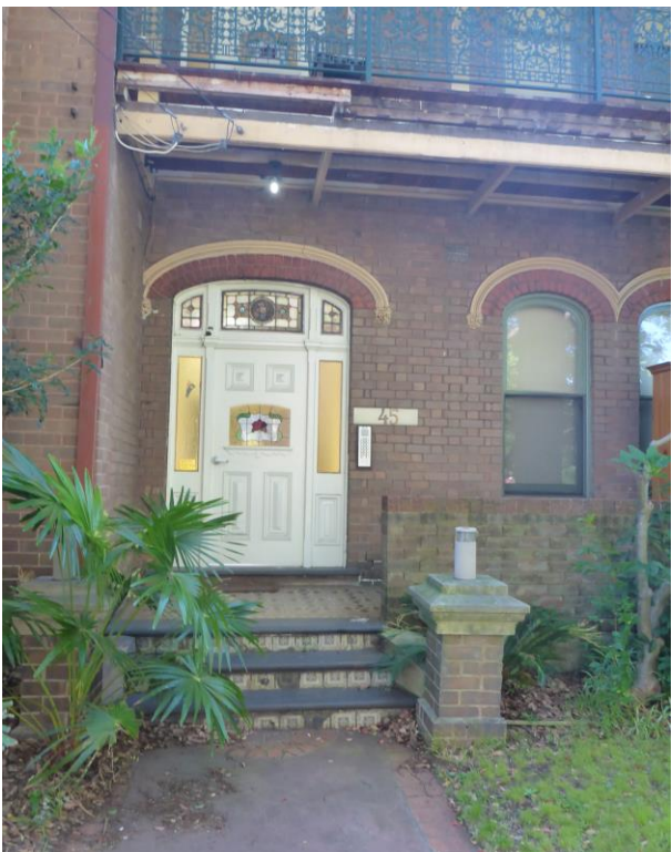
PICTURE 17 – DETAIL LOWER GROUND LEVEL FRONT FAÇADE.
