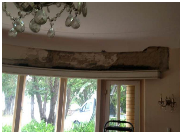
PICTURE 23 – INTERIOR OF CURVED FRONT SECTION OF THE HOUSE
