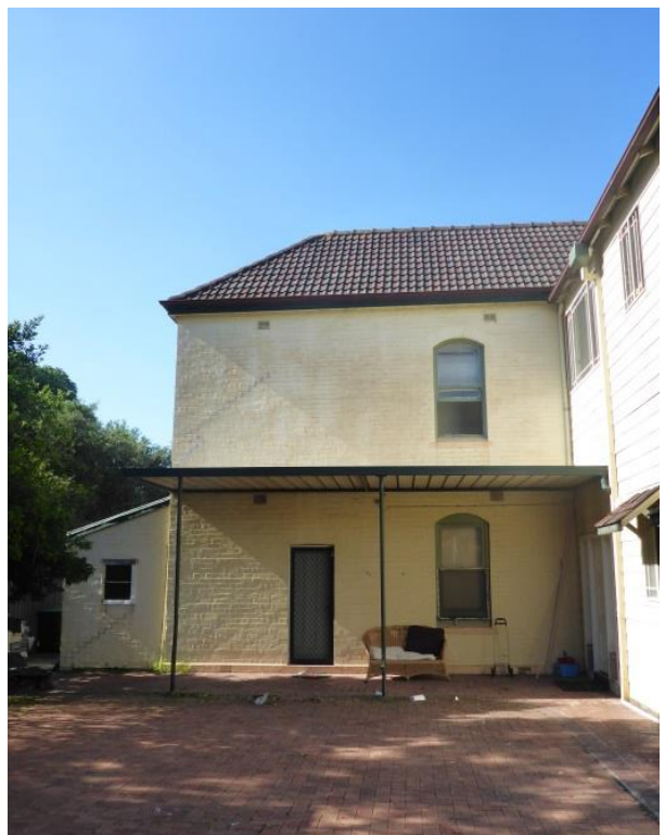
PICTURE 18 – NORTHERN FAÇADE.
