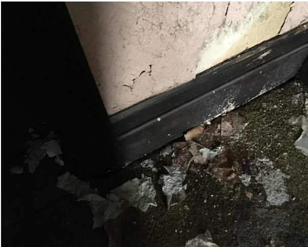
PICTURE 9 – INTERNAL VIEW OF SKIRTING.
