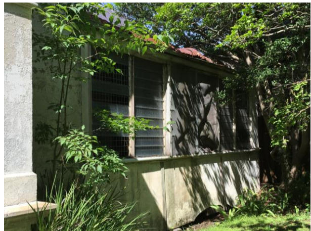
PICTURE 2 – EXTERNAL VIEW OF INFILLED WESTERN FAÇADE.
